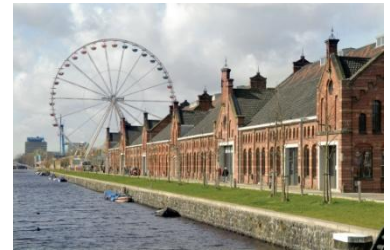
fig. 10_Wastergas Fabriek - Waterfront public space
